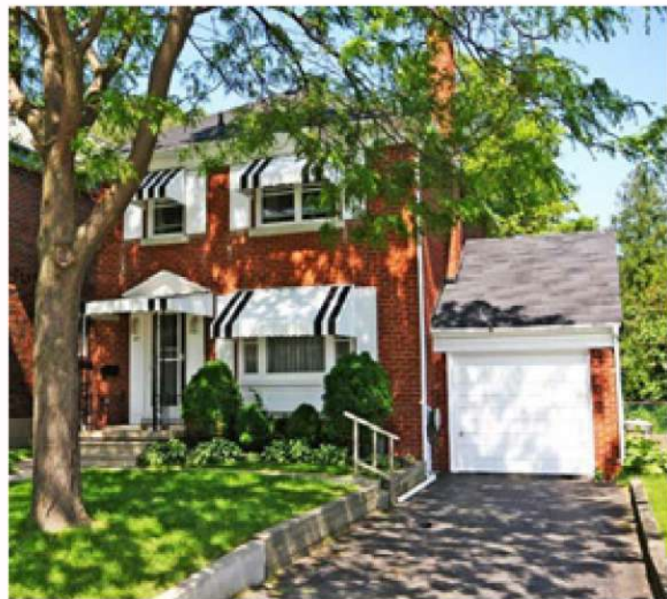
Simply put: 33 Kelso before the complete home renovation.
